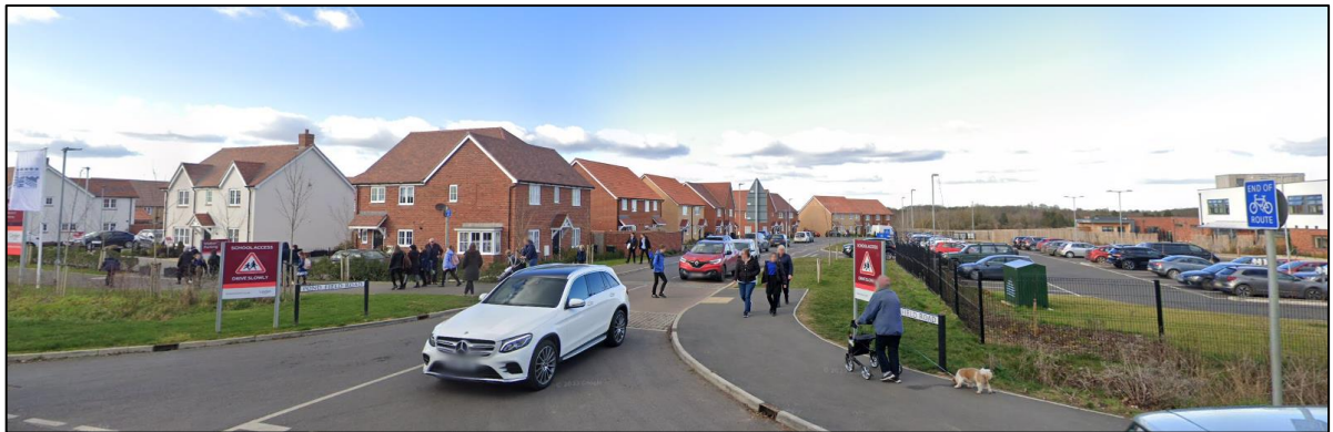
figures 21: The well-used footway/cycleway provided by Linden homes on the site frontage to the Cavendish View development
